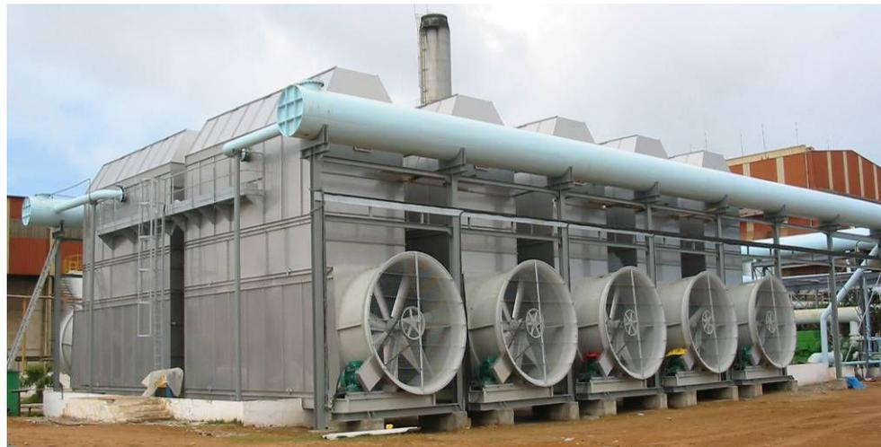
Flow rates : from 70 to 660 m<sup>3</sup>/ h/cell
